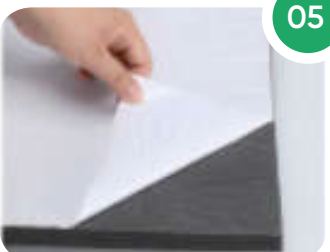
05 Peel off the backing paper Do not touch the backing adhesive with your hands which will affect the stickiness
