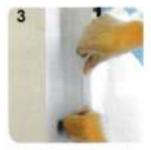
First stick the wide side A (zipper is closed) with the open window from the middle to the left and right side or to the up and down side to the window frame.
