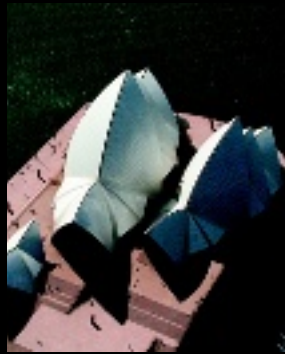
The three groups of interlocking shells are set on a vast terraced platform. © Michael Moy Idea to Icon
