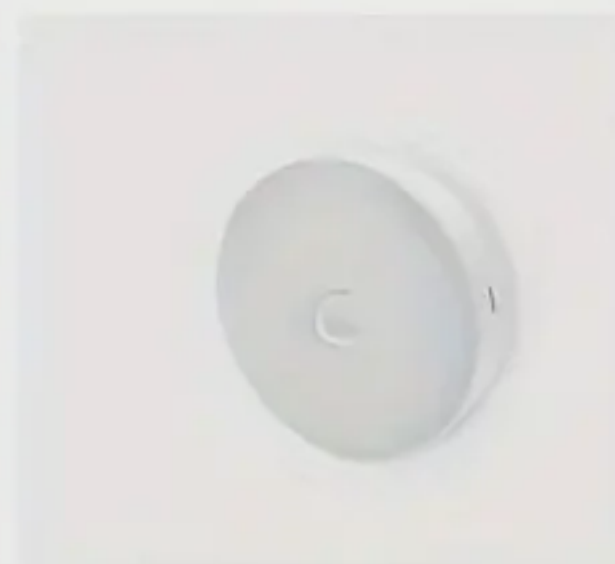
6. The installation is complete
