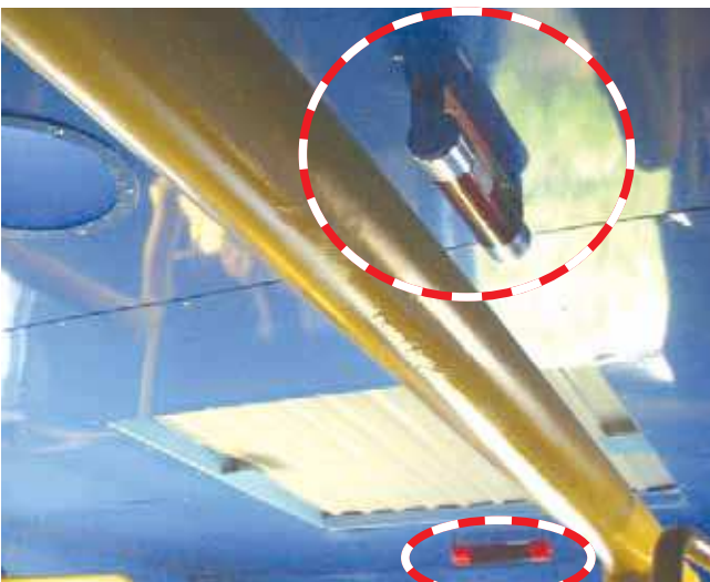
Implementation of the ampoule BONPET engine room ceiling
