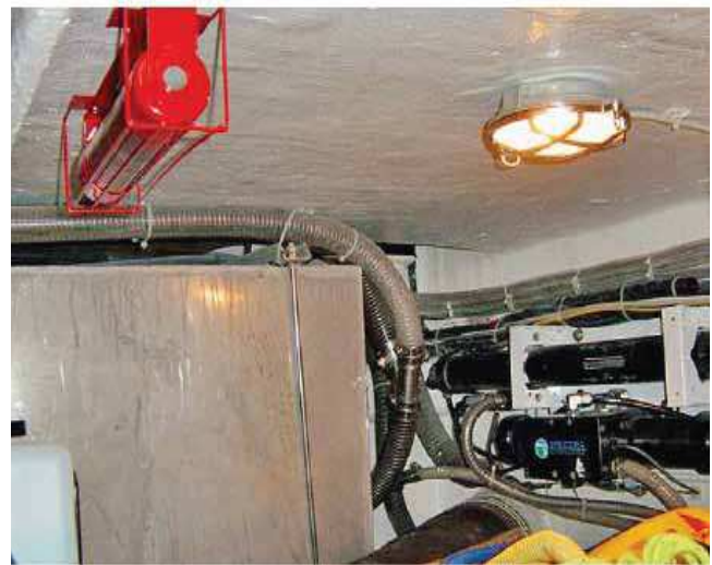
Implementation of the ampoule BONPET near electronic equipment that is impossible to meet with systymata whole sprawling
