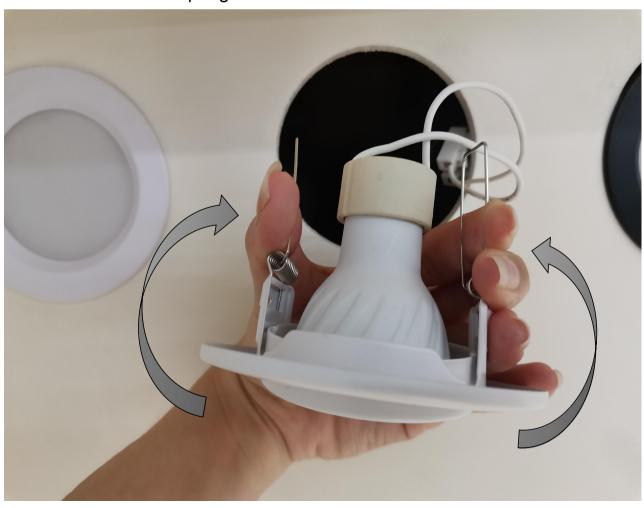
10. Put both springs into the hole in the ceiling and release.
