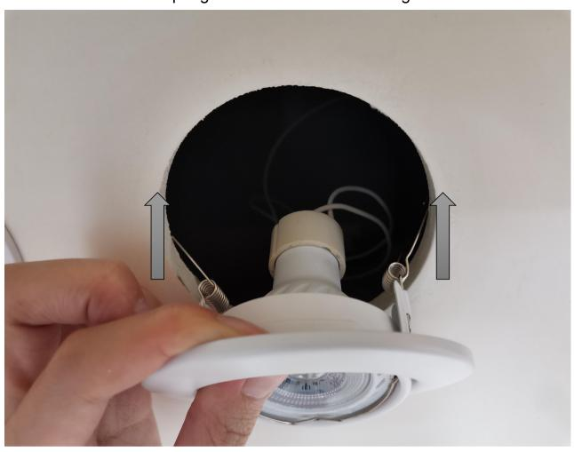
11. Adjust the inner ring to the desired Angle and energize.
