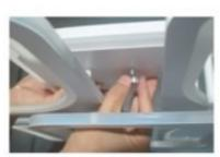
lift up the light and install it to the hanger, the four flat-headed screws go through the plate, and fasten with the nuts as shown
