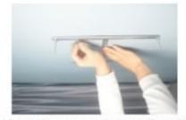
12, install the hanger to the ceiling with sharp pointed screws using a electric drill do not move the flat-headed screws
