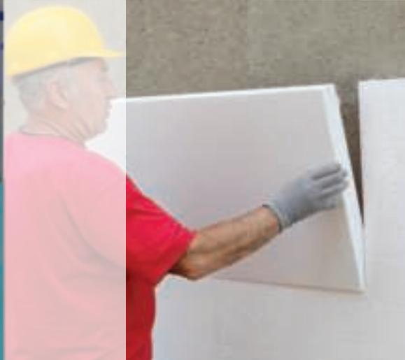
Apel Adhesive Foam is a polyurethane based, single componenet, moisture curing gun-foam that is used to bond styrofoam, XPS, EPS insulation panels.
