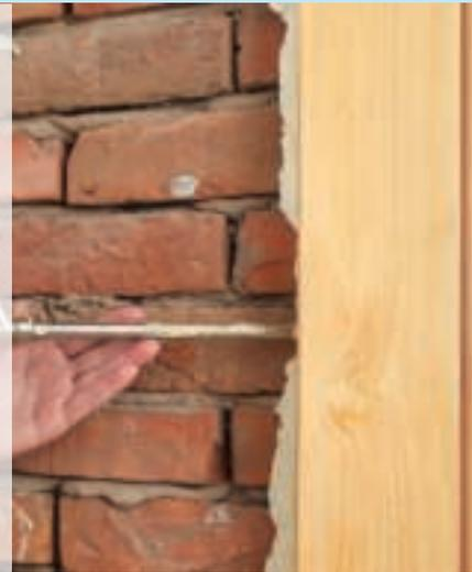
Apel PU Professional Foam (Gun Foam) is a single component, moisture curing, insulation and installation foam. It is applicable with a foam-gun for installing door and window frames in construction industry.
