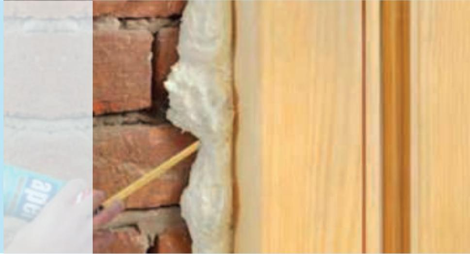
Apel Safety Valved Foam is a polyurethane based, single component, moisture-curing, installation and insulation foam which is used in fixing door and window frames on constructions.
