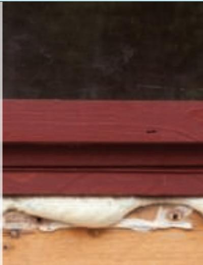
Apel PU Foam is a polyurethane based installation and insulation foam which is used in fixing door and window frames in constructions. Excellent expansion and gap filling properties and solid rigid form after curing make the foam choice of professionals.
