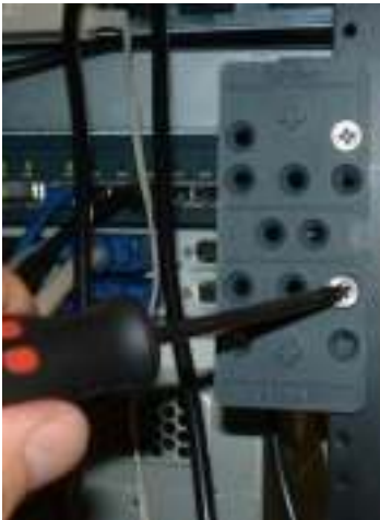
Figure D-2 Attaching the Mounting Bracket
