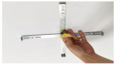
11, install the cross with the screws to th ceiling
