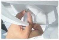
11, lift up the light and install it to the cross, the four flat-headed screws go through the plate, and fasten with the nuts as shown
