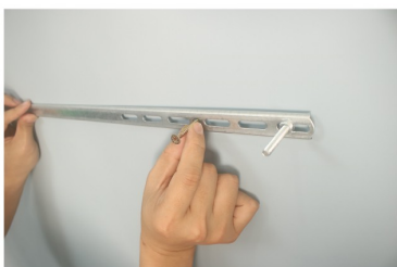
7, install the hanger with the sharp point screws to the ceiling
