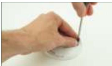
Screw the bottom plate tight on the ceiling. Make sure that the bottom plate is tight against the ceiling so no air can circulate above the smoke detector and impede smoke detection. If necessary seal this opening with mastic.
