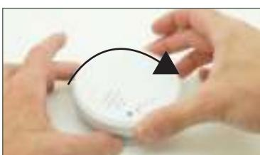
Fit the smoke detector on the bottom plate and turn it clockwise (to the right).
