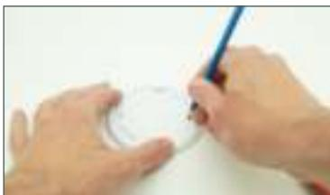
Use a pencil to mark the drill holes through the mounting bracket on your ceiling. Drill the holes and insert the plugs if necessary.
