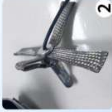
Fold the copper strips if needed
