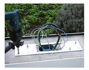
c. Mount the floor plate over the anchors and make sure it is level in both directions. If not, tilt the floor plate until it becomes level.
