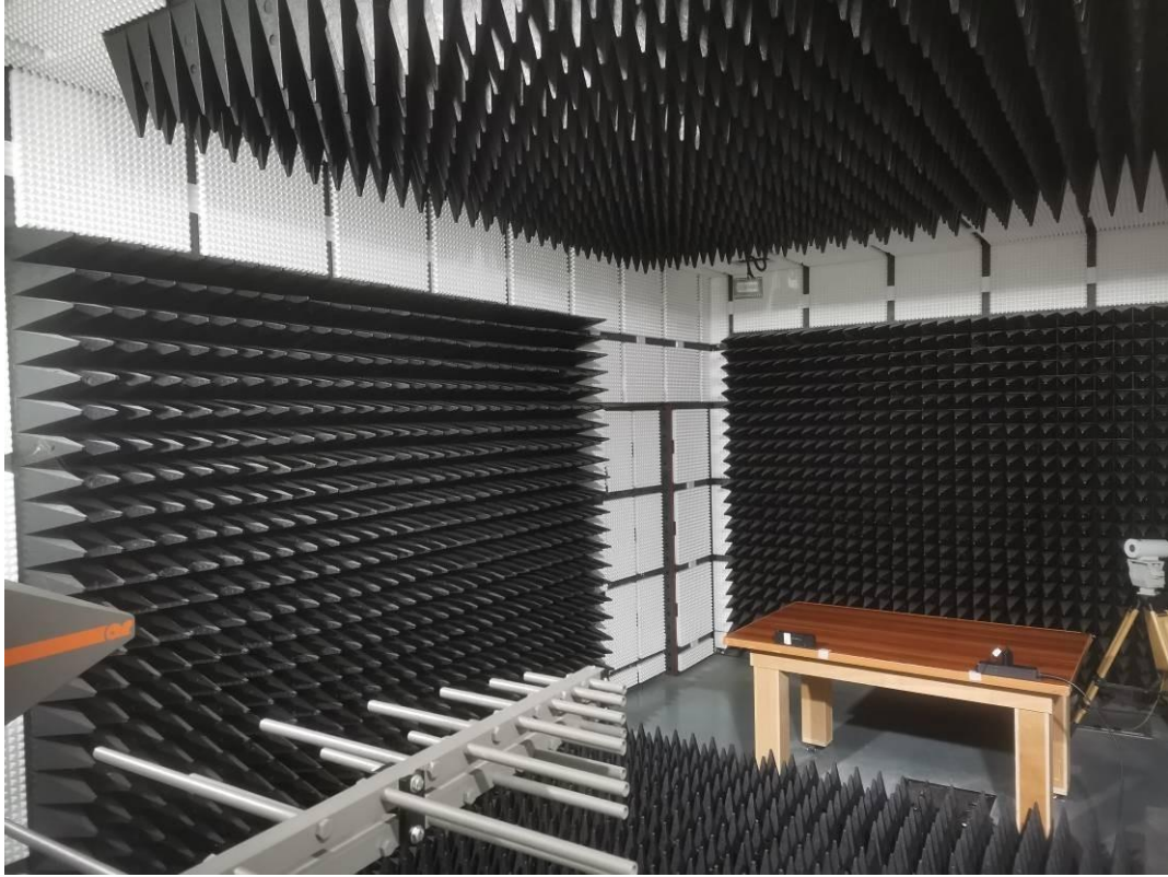
Test Setup Photo View
