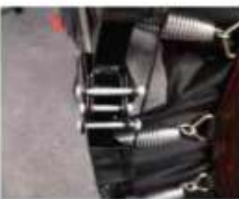
13 Mounting the screws of the handrail
