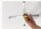
8. install the cross with the sharp-ended screws to the ceiling (the flat side of the cross should be faced to the ceiling)
