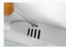
9. connect the wires of the light to the home electric system, and install the light to the cross with the screws
