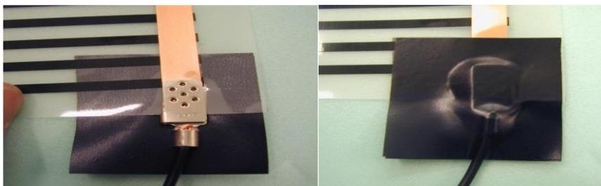
**After installation CAUTION:** Always insulate the shrink connectors by cutting 2 pieces of insulating tape and sticking them on both sides over the shrink connectors. The tape must be fixed at least 5 mm over the end of the shrink connector. The end of the underfloor heating foil must also be insulated with insulation tape.
