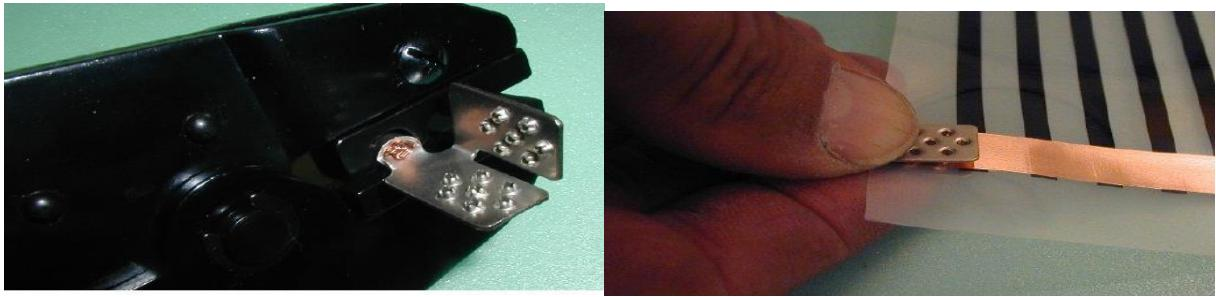
Once the entire floor area is covered with the Quality Heating underfloor heating foil, the power wires may be connected. Clamp the shrink connector using the pressure distribution pliers / shrink pliers (picture above). Pay attention with a single power wire, (1st connection) always double fold the core wire! Always squeeze both sides of the connector to the wire. Then place the shrink connector over the copper conductor on the heating foil. Squeeze the pressure distribution pliers tightly.
