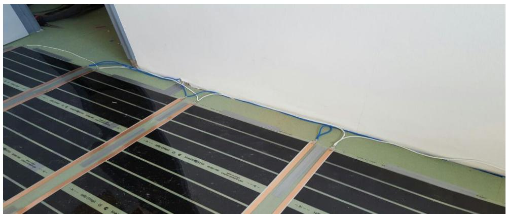
Make two slots in the wall from the point where the thermostat is mounted to the floor. One tube contains the connecting wires of the underfloor heating foil and the other tube contains the 'sensor, floor sensor'.
