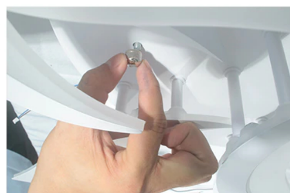
15: Life up the light and install it to the cross, the four flat headed screws go through the plate and then use the nuts to fasten the light.
