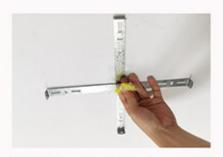
8, install the cross with the sharp-ended screws to th ceiling (the flat side of the cross should be faced to the ceiling)
