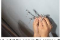
12, install the cross to the ceiling with sharp pointed screws using a electric drill do not move the flat-headed screws
