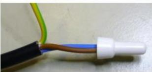
Twist the wires together along the entire lengths of the scrip.
